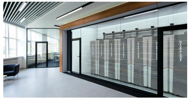
With the scalable and made to measure Hydraloop Cascade system, you can recycle up to 95% of shower, bath and/or handbasin water + the cooling water from air-conditioning units. Due to its innovative and breakthrough technology the maintenance requirements and corresponding costs are very low.
