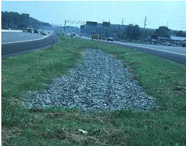
**Description:** Infiltration practices are designed and constructed to capture and treat stormwater runoff through:
