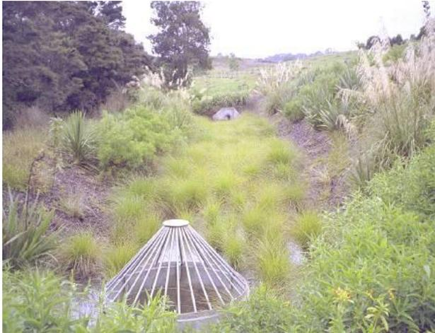
**Description:** Wetlands are designed and constructed to capture and treat stormwater runoff through:
