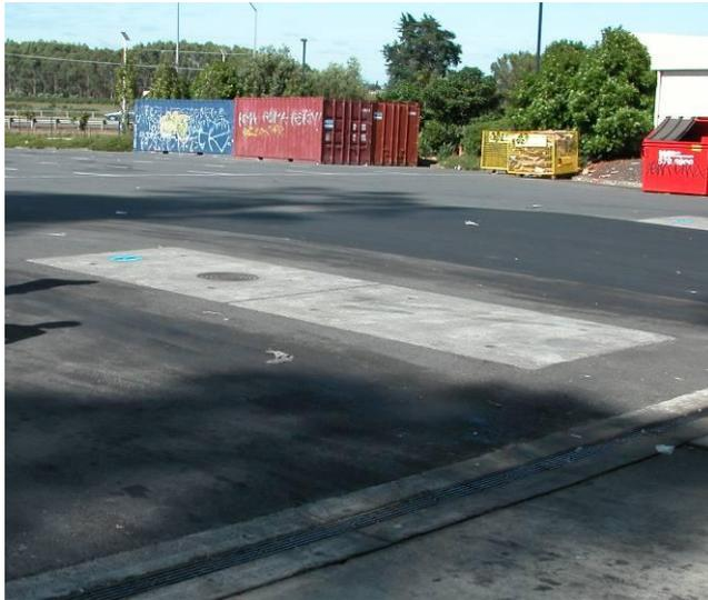
Oil water separator devices are applicable for treating stormwater runoff from areas where hydrocarbon products are handled or where hydrocarbon loads can be very high. They should be located as close to the source of the hydrocarbons as possible to retain the oil in a floatable, non-emulsified form.
