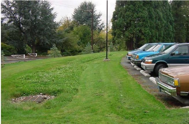
**Description:** Filter strips are uniformly graded and densely vegetated to treat stormwater runoff by the following:
