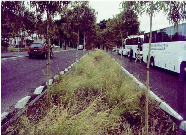
**Description:** Rain gardens are designed and constructed to capture and treat stormwater runoff through:
