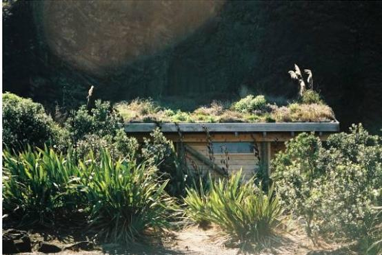
**Description:** Green roofs are roofs with a growing media that reduces stormwater runoff through evaporation and evapotranspiration. Their primary benefit from a stormwater management perspective is to reduce the total volume of stormwater runoff.
