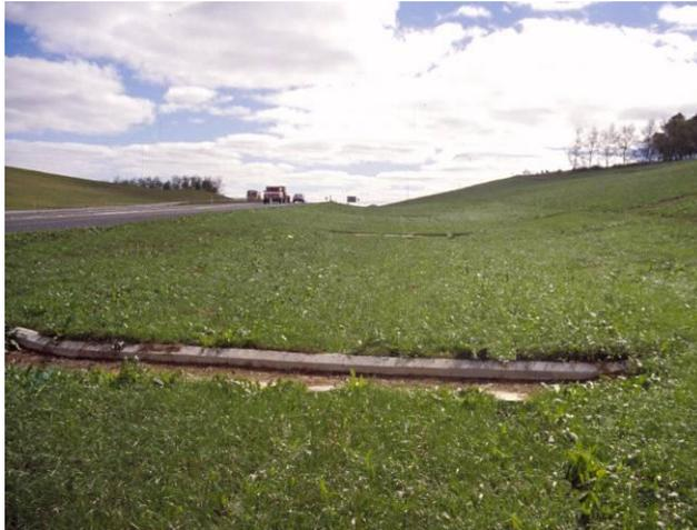
**Description:** Vegetated swales are designed and constructed to capture and treat stormwater runoff through:
