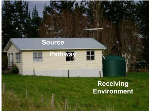
**Description:** Water tanks provide detention storage for stormwater runoff and water supply for domestic use. They reduce stormwater runoff through domestic use and thus reduce the total volume of stormwater being discharged during a storm event.
